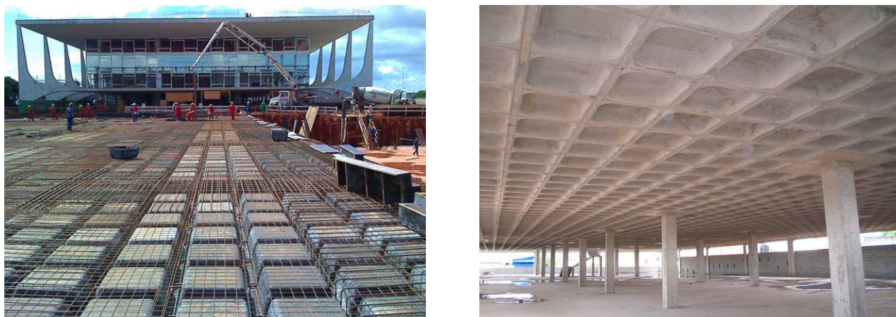
Figura 67 – Laje nervurada com moldes plásticos. ( http://www.flickr.com/photos/atex ).
